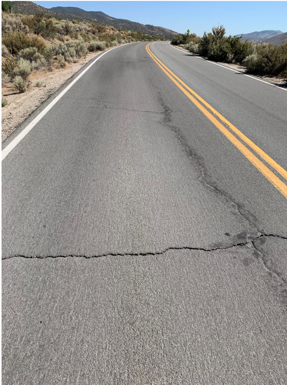
Figure 4. Pavement in Fair condition category (PCI 70-56).
