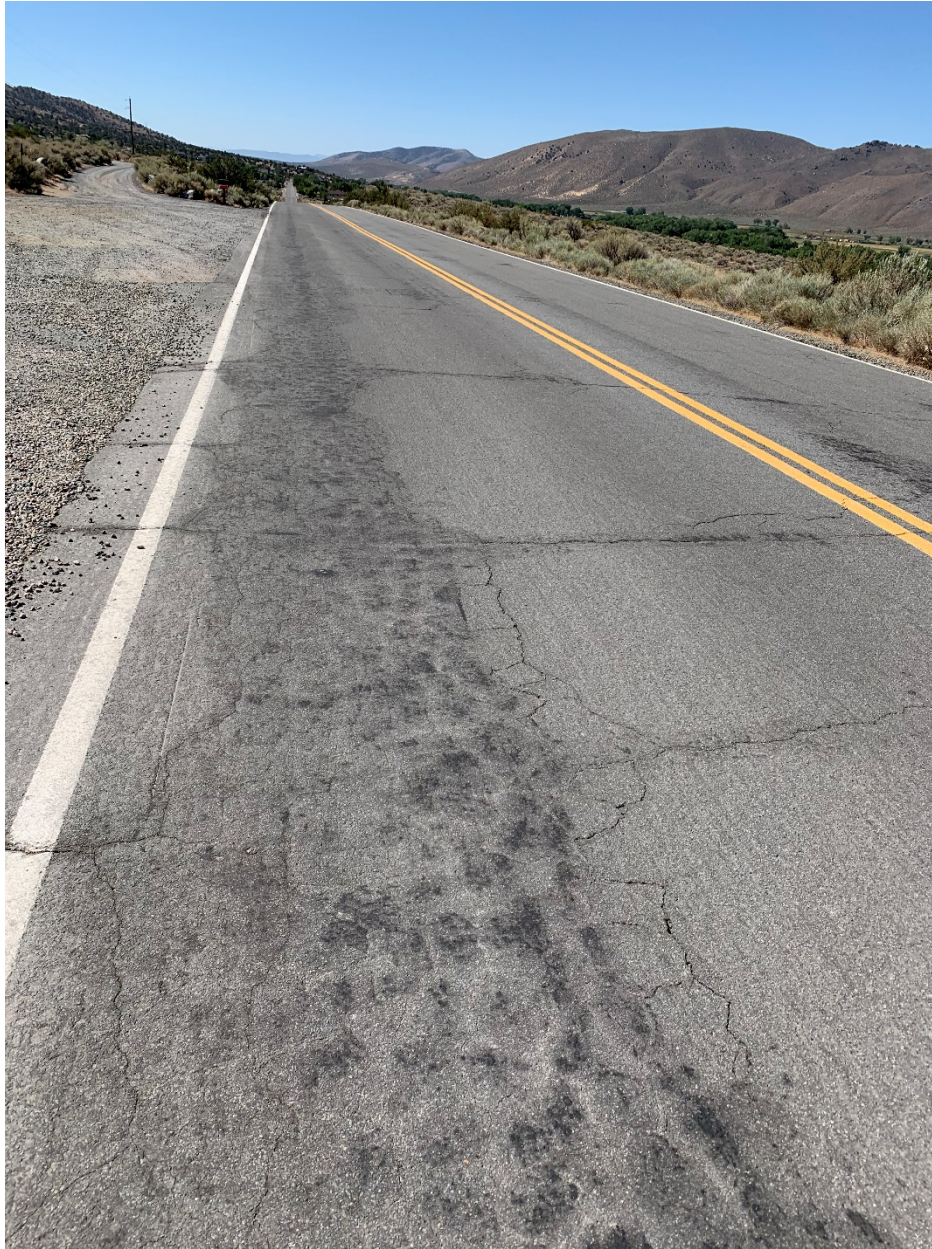
Figure 7. Pavement in Serious condition category (PCI 25-11).
