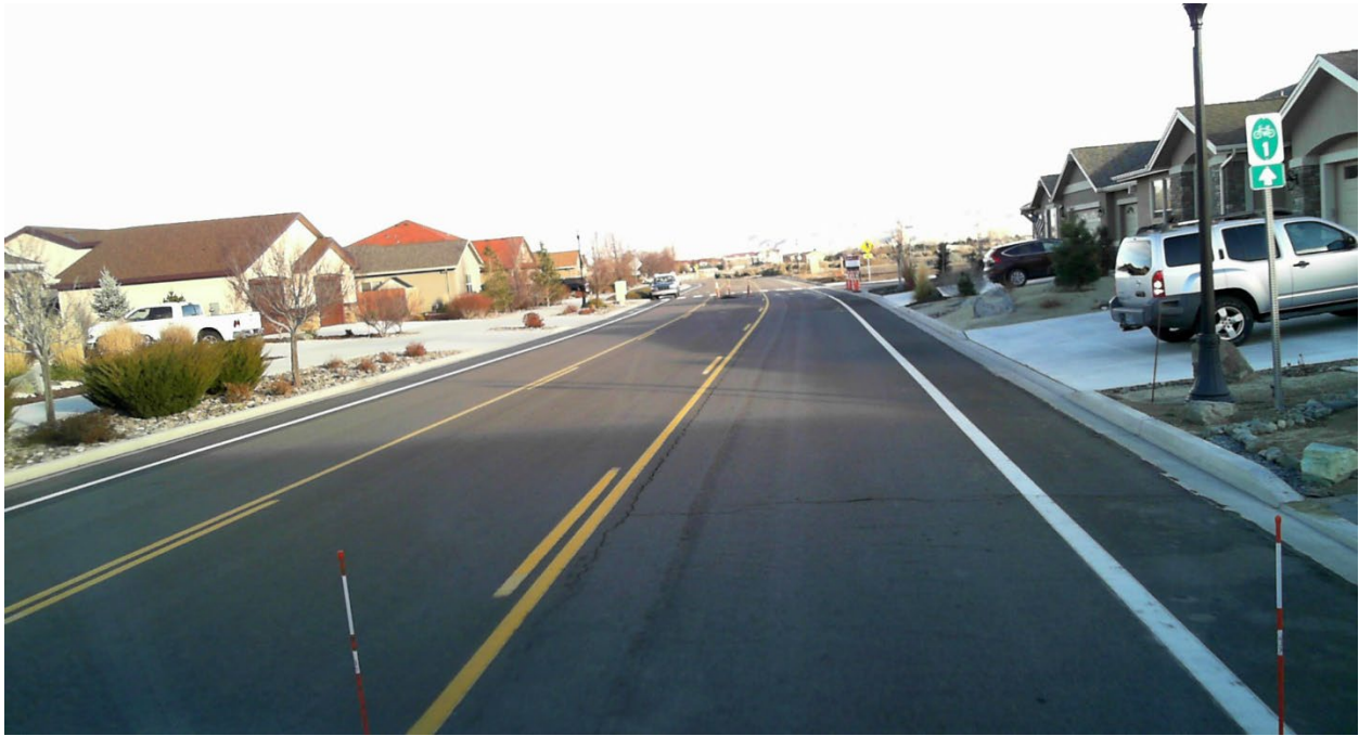
Figure 3. Pavement in Satisfactory condition category (PCI 85-71).
