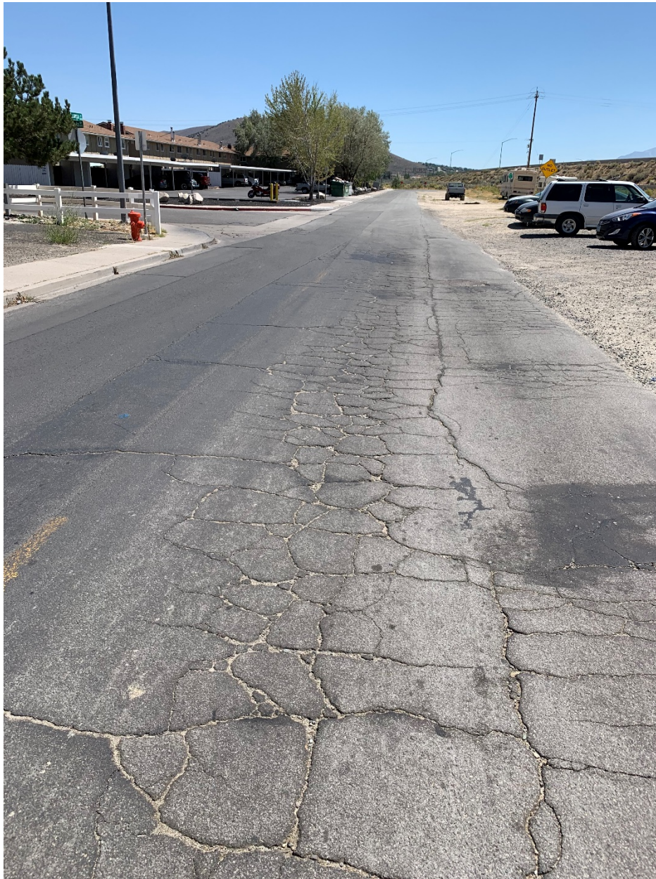
Figure 6. Pavement in Very Poor condition category (PCI 40-26).
