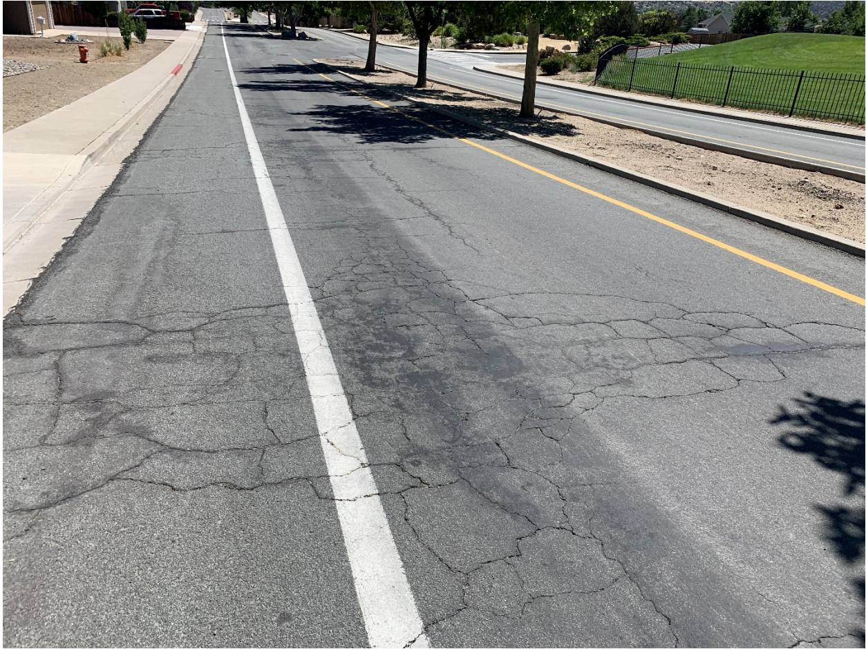
Figure 5. Pavement in Poor condition category (PCI 55-41).
