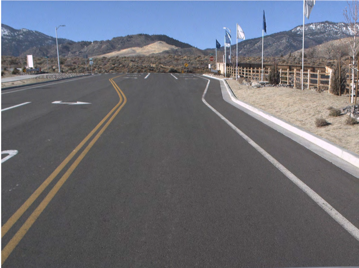
Figure 2. Pavement in Good condition category (PCI 100-86).
