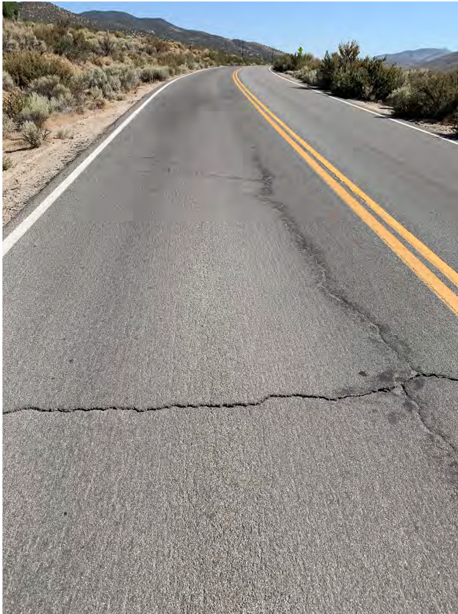
Figure 4. Pavement in Fair condition category (PCI 70-56).
