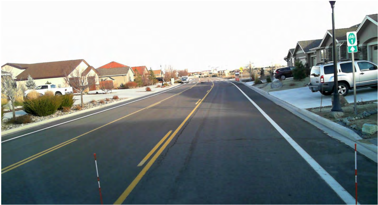
Figure 3. Pavement in Satisfactory condition category (PCI 85-71).
